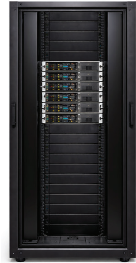
Day 1: Initial CPU Installation
