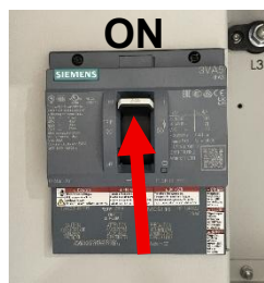
Figure 27—AC main power switch in ON position and LCD display of current power level
