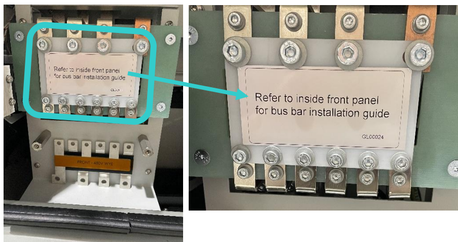
Figure 15— White plastic spacer plate secured to Bus Bar to be replaced with a Configuration Bus Bar
