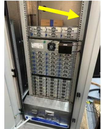
Figure 6 – Open area above power stacks of 120 kW fast charger or 60 kW bi-directional charger (shown here) provides access to back side of charger's front wall
