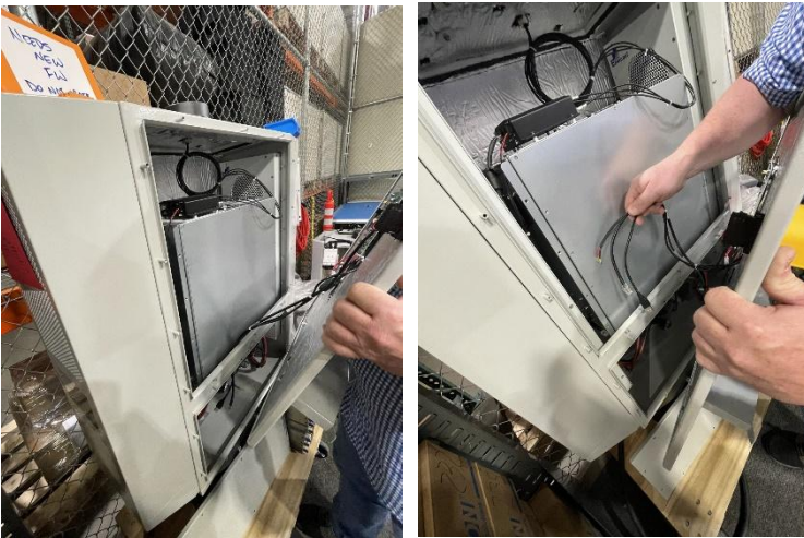
Figure 13: Guide cables out from behind charger's front bracket
