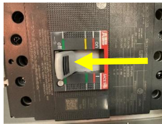
Figure 3: 30 kW charger's AC Main Switch inside charger in OFF position
