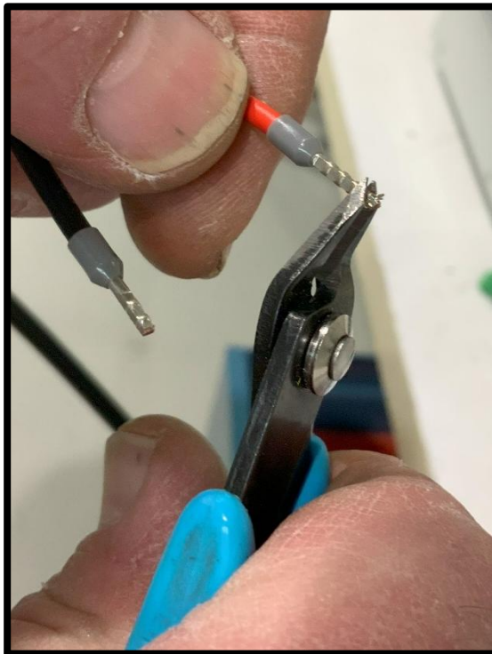
Figure 11 – Trimming wire ferrules of enclosed cable
