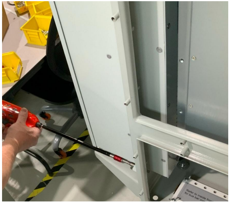
Figure 8 – Removing 20 fasteners
