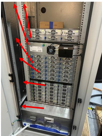
Figure 10 – Left-side door grants access to 6 of the 12 M6 bolts that secure HX to charger's back wall
