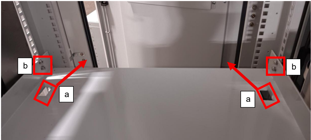
Figure 19 – Shelf for HX power source installed
