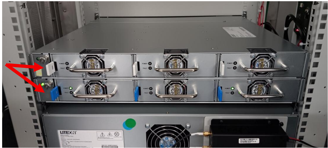
Figure 8 – Heat Exchanger power source installed above Rack Controller in
