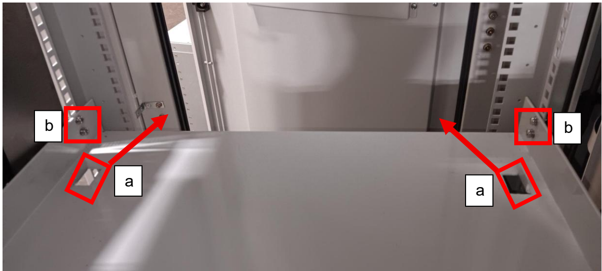
Figure 15 – Shelf that supports installed HX power
