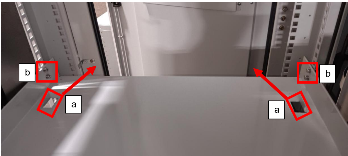
Figure 22 – Shelf for HX power source installed
