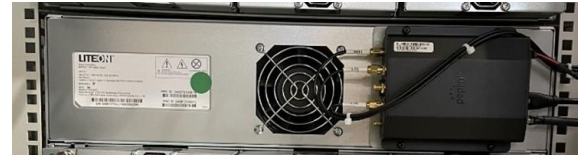
Figure 10 – Front of installed rack controller with modem still attached
