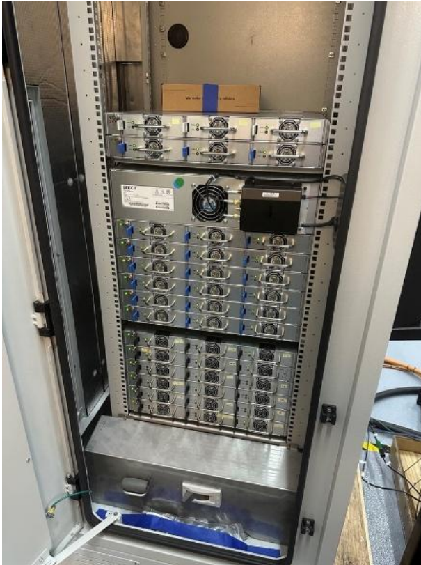
Figure 2: Inside left-side door of 60 kW Bi-Directional Charger with modem secured to installed rack
