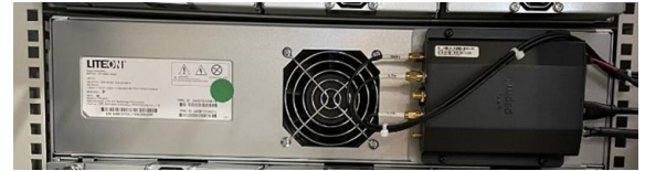
Figure 10 – Front of installed rack controller with modem still attached
