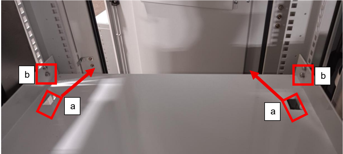
Figure 19 – Shelf for HX power source installed
