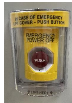
Figure 49 –Pressing Emergency Power Off button is only for Emergencies. DO NOT press to stop a normal charging session.
