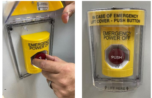
Figure 53 - Reset Emergency Power Off button
