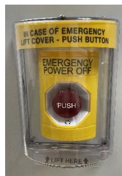
Figure 48 –Pressing Emergency Power Off button is only for Emergencies. DO NOT press to stop a normal charging session.
