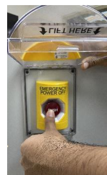
Figure 48 –Pressing Emergency Power Off button is only for Emergencies. DO NOT press to stop a normal charging session.
