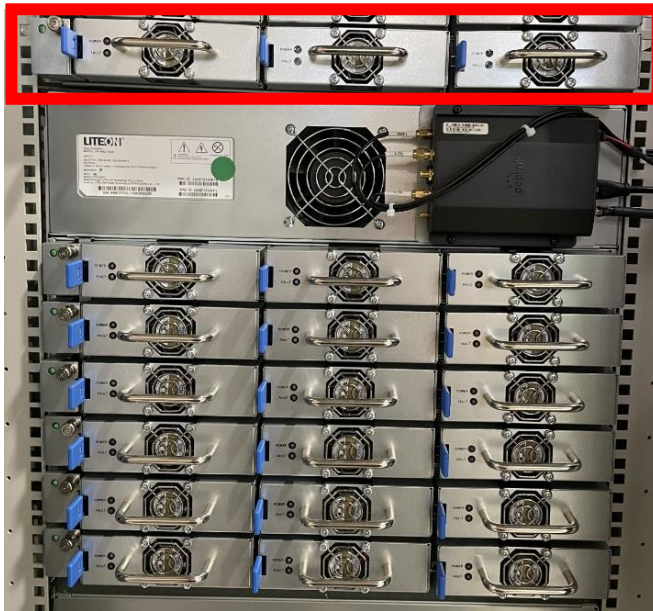
Figure 31—Three uniquely identified Rectifier modules (tab color may differ) are reserved for the top shelf and will provide power to the Heat Exchanger
