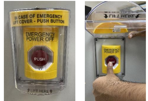
Figure 49 – Pressing Emergency Power Off button is only for Emergencies. DO NOT press to stop a normal charging session.
