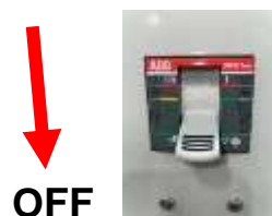
Figure 4—AC main power switch in the OFF position
