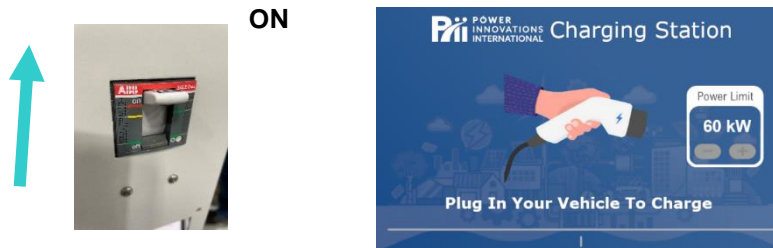
Figure 23—AC main power switch in ON position and LCD display of current power level
