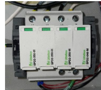
Figure 31 - SPD with four green modules
