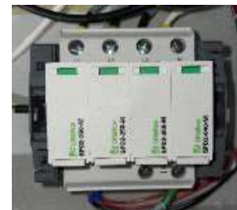
Figure 36—SPD with four green modules
