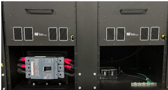
Figure 6—From left to right: Breaker, Terminal Block, Ground Bus Bar, and Sample Terminal Block Configuration
